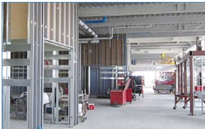
Laboratory space under construction
