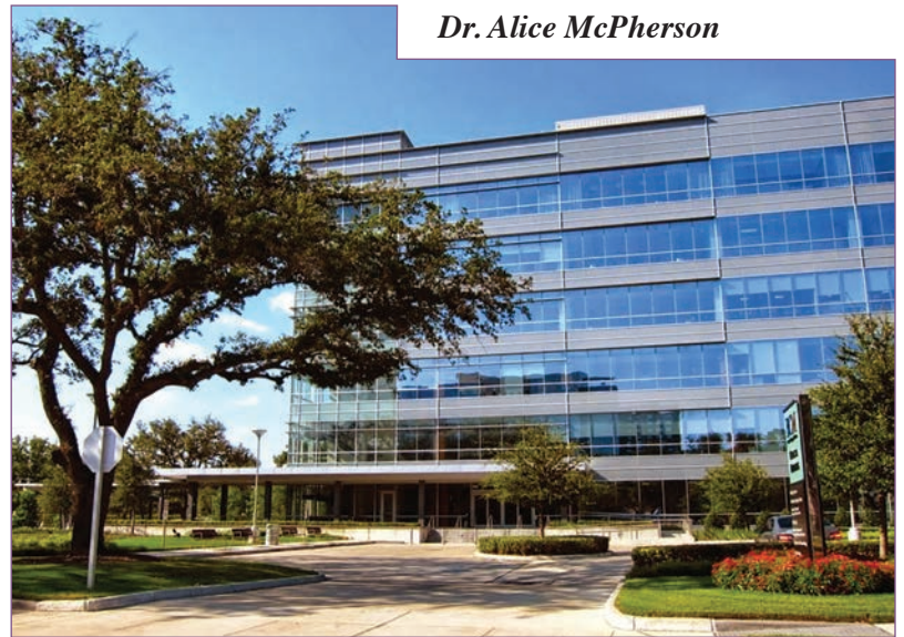
Retina Research Foundation Headquarters, 4th Floor, Houston, Texas.
